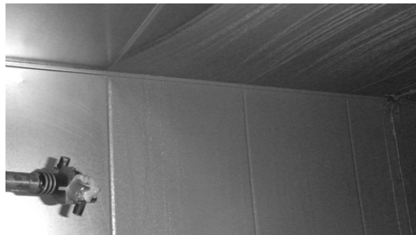
Figure 4.10: Class A robotic application of sealant.
